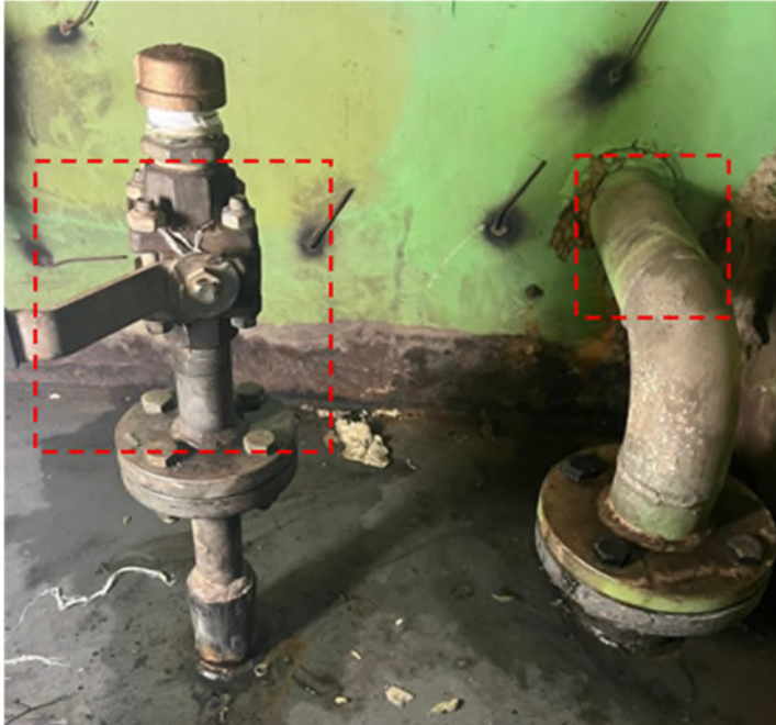
Flanged connection for level transmitter near corroded M4 ventilation pipe (to atmosphere)
