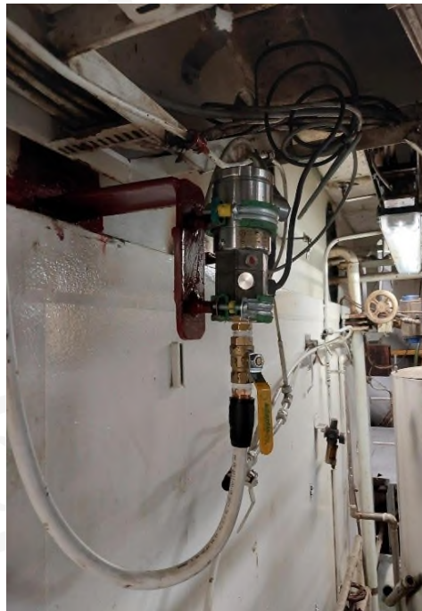
First stage (left) and second stage (right) level transmitter for tank M4, relocated outside of access space
