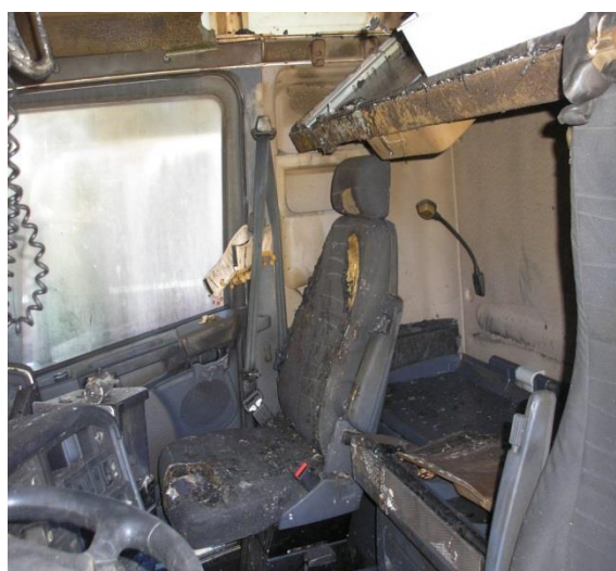
Photograph No. 15. Burnt driver's cabin of the refrigerator truck
