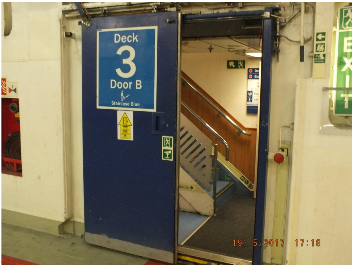
Photograph No. 42. Automatically closed door dividing the car deck from the staircase to passenger rooms
