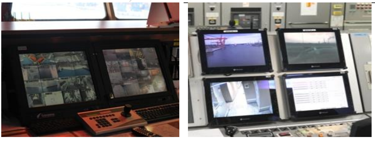
Photograph No. 26. CCTV images on the screens on the bridge (left) and in the engine control room (right)
