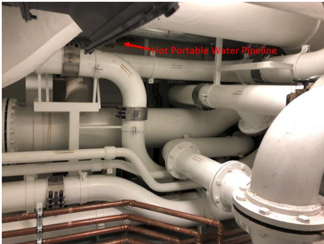
Figure 4: Location of hot potable water pipeline where leakage was observed
