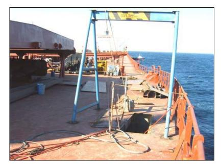
Access was cut through the deck of the vessel in order to position and weld the new steel in place, photograph taken on the port side of cargo hold No.1
