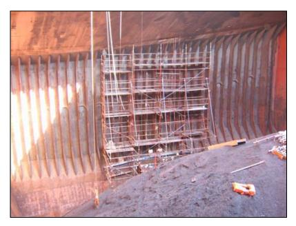
Cargo hold No.1, Port side, frames 312 and 313, temporary repairs in progress, new steel welded to badly corroded / wasted frames.
