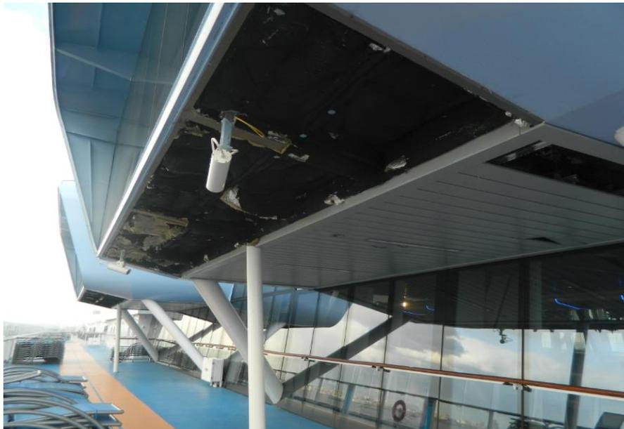
**Figure 14: Damaged ceiling on deck**
