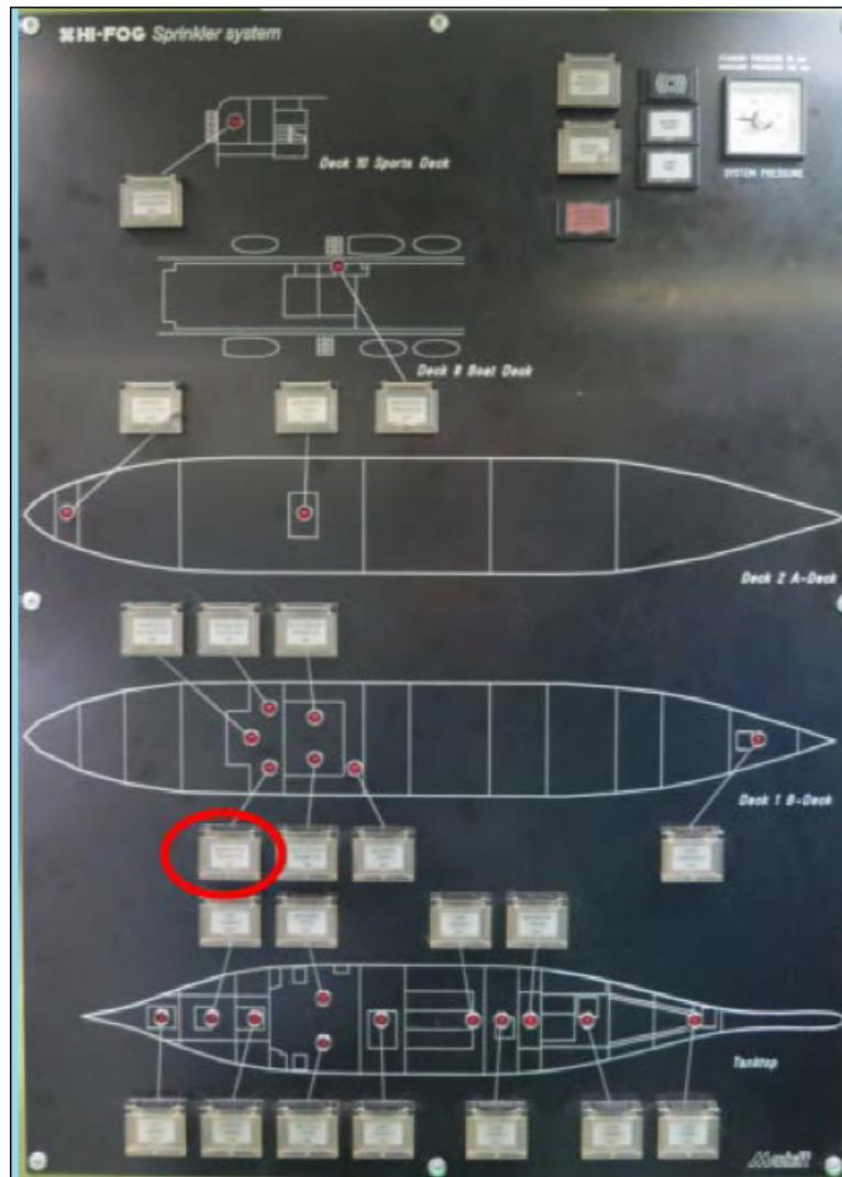
Figure 7: Hi Fog Control Panel
