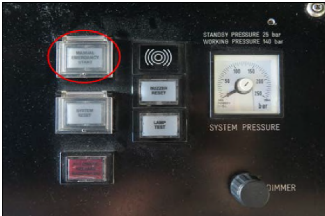
Figure 21: Bridge – Emergency Start Button
