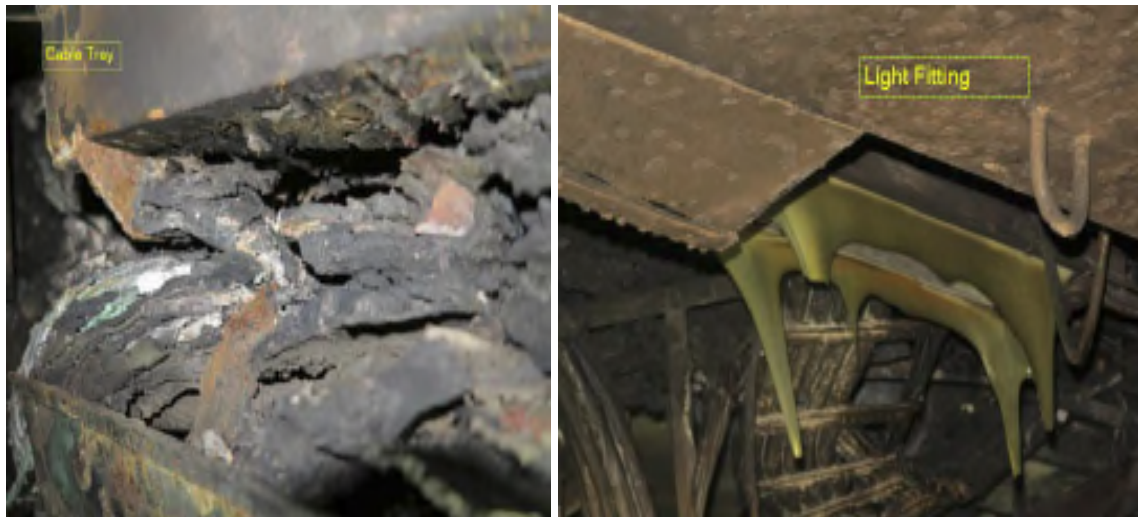
Figure 14: Collateral damage to cable tray (left) and light fixture in vicinity of AE1 (right)
