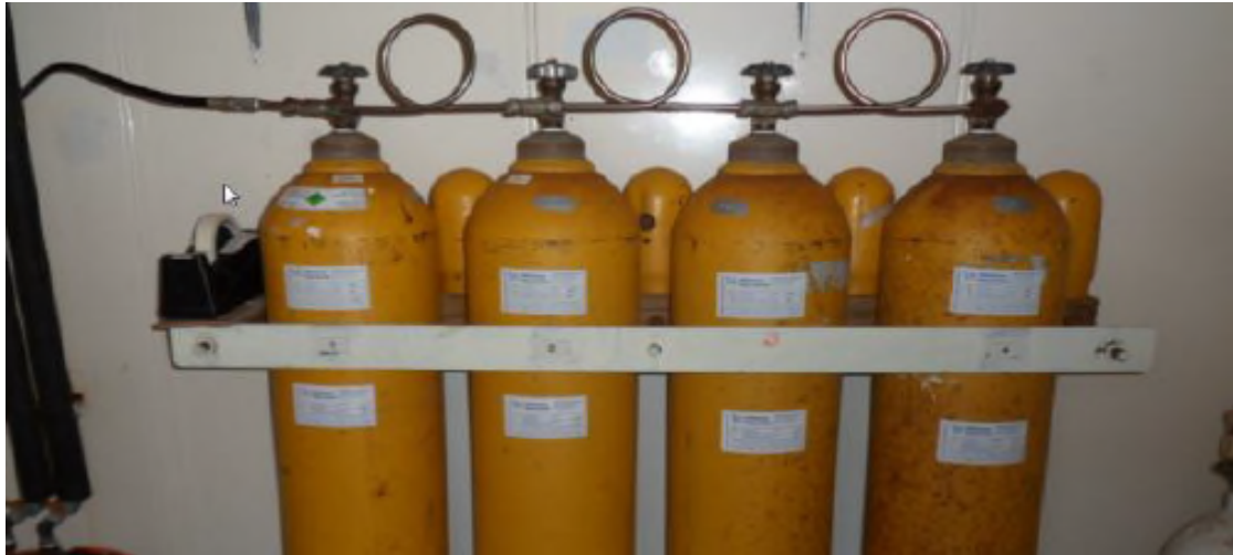
Figure 21: BA compressor cascade system and below 6-litre BA bottles
