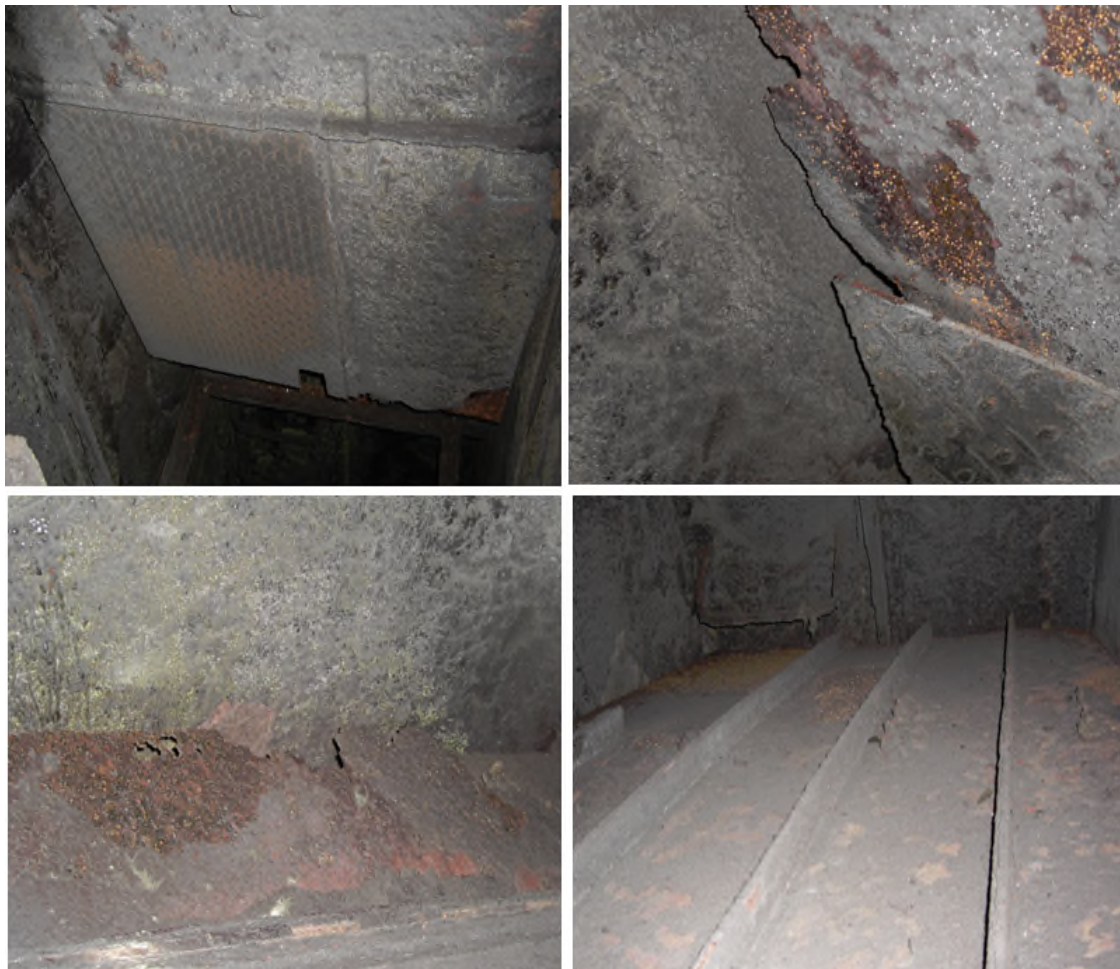
Figure 26: Auxiliary engine room fire dampers
