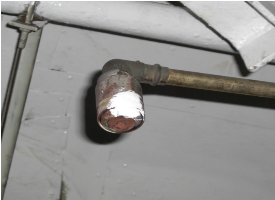
Figure 17: Damaged nozzle located in vicinity of auxiliary generators 4 and 5
