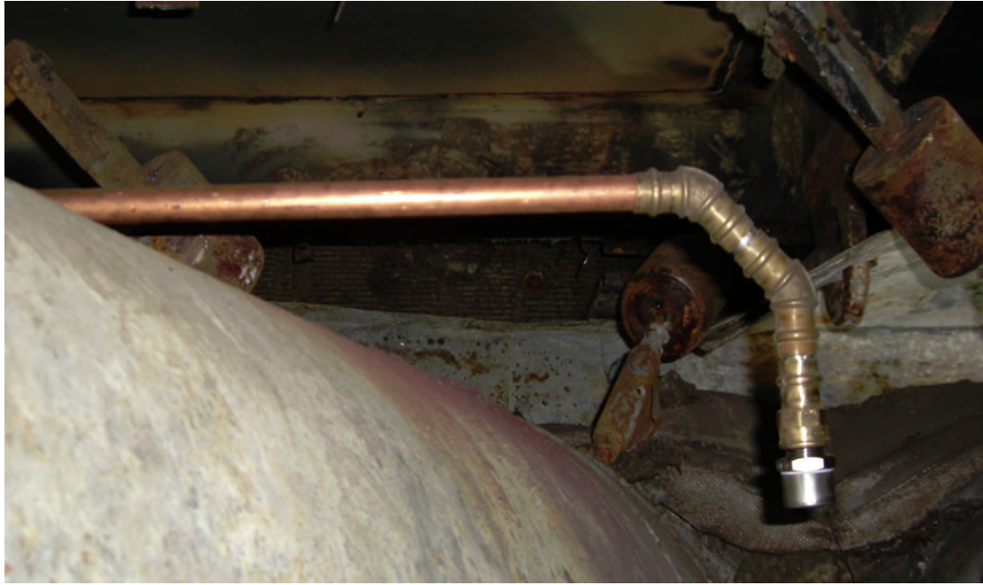
Figure 24: Copper pipe used to rectify flexi-fog piping after the fire
