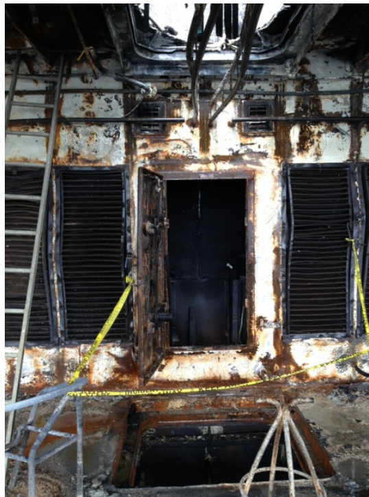
Aluminium hatches destroyed in fire
