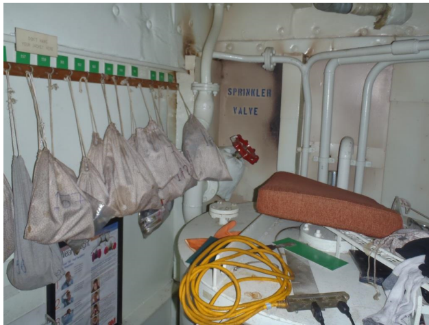
8 General View in Bosun's Workshop on Deck No. 3 Aft (Note the location of the aft mooring deck fire suppression system valve)
