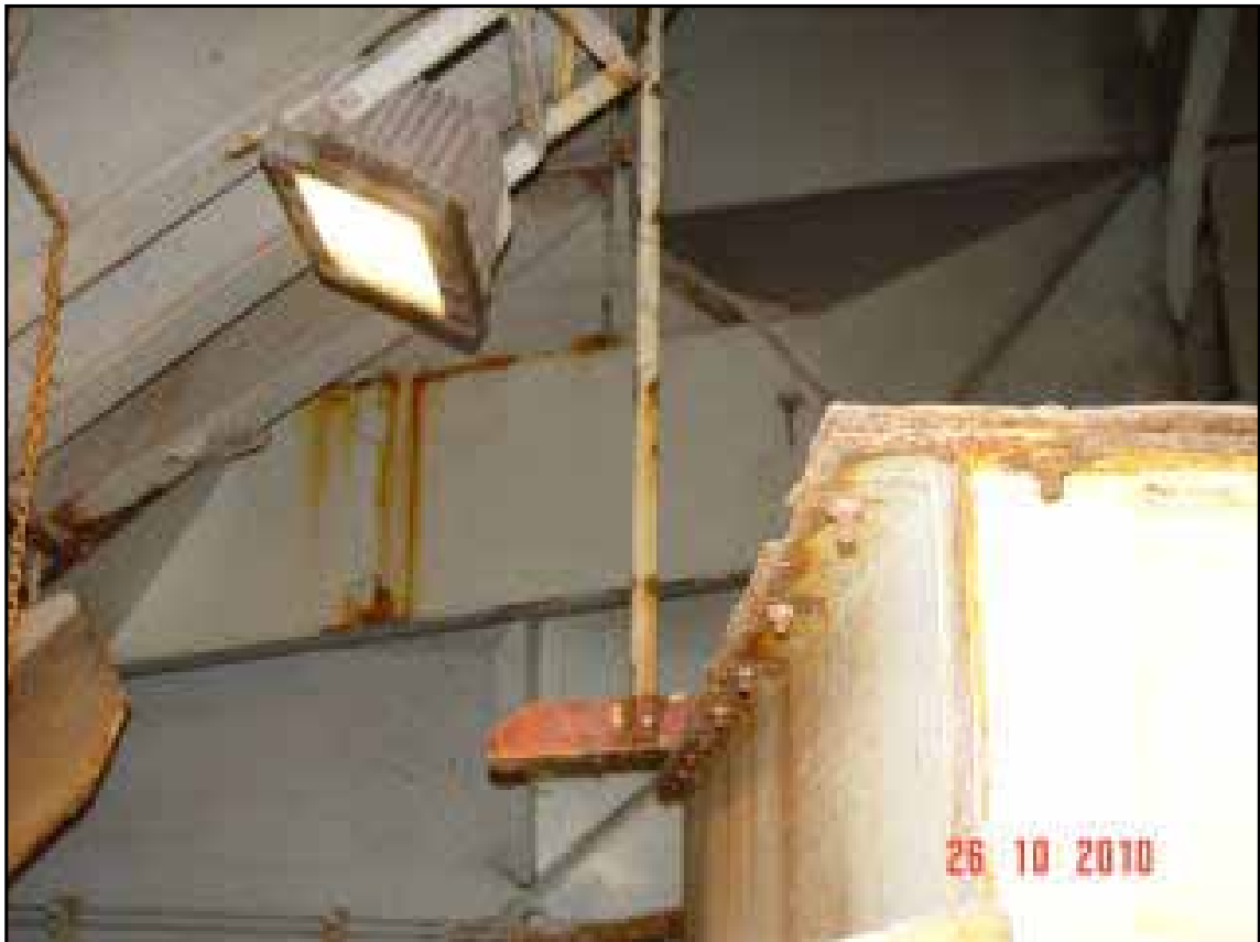
500W halogen lamp fitted to Yeoman Bridge
