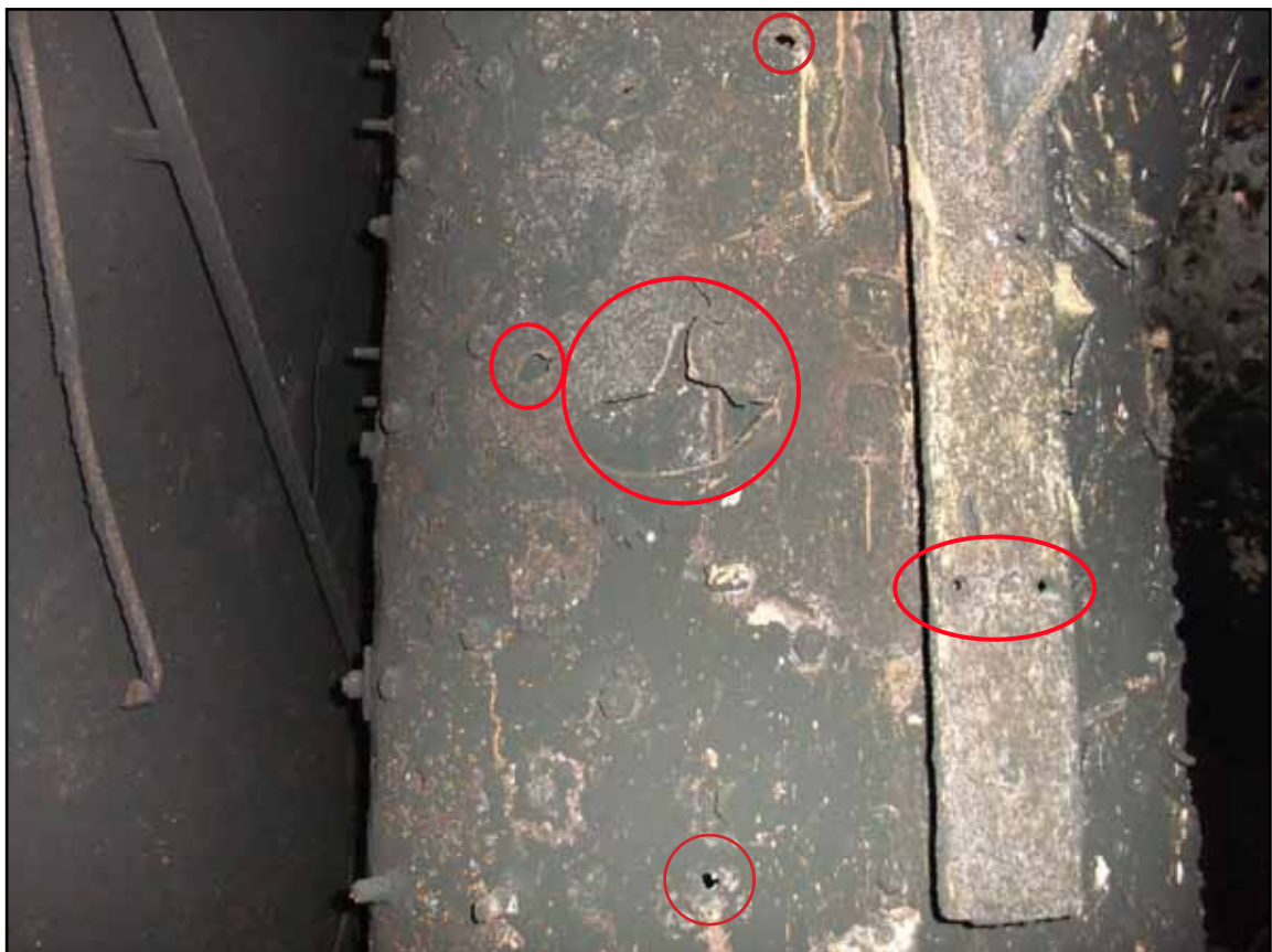
Hopper carcass penetrations
