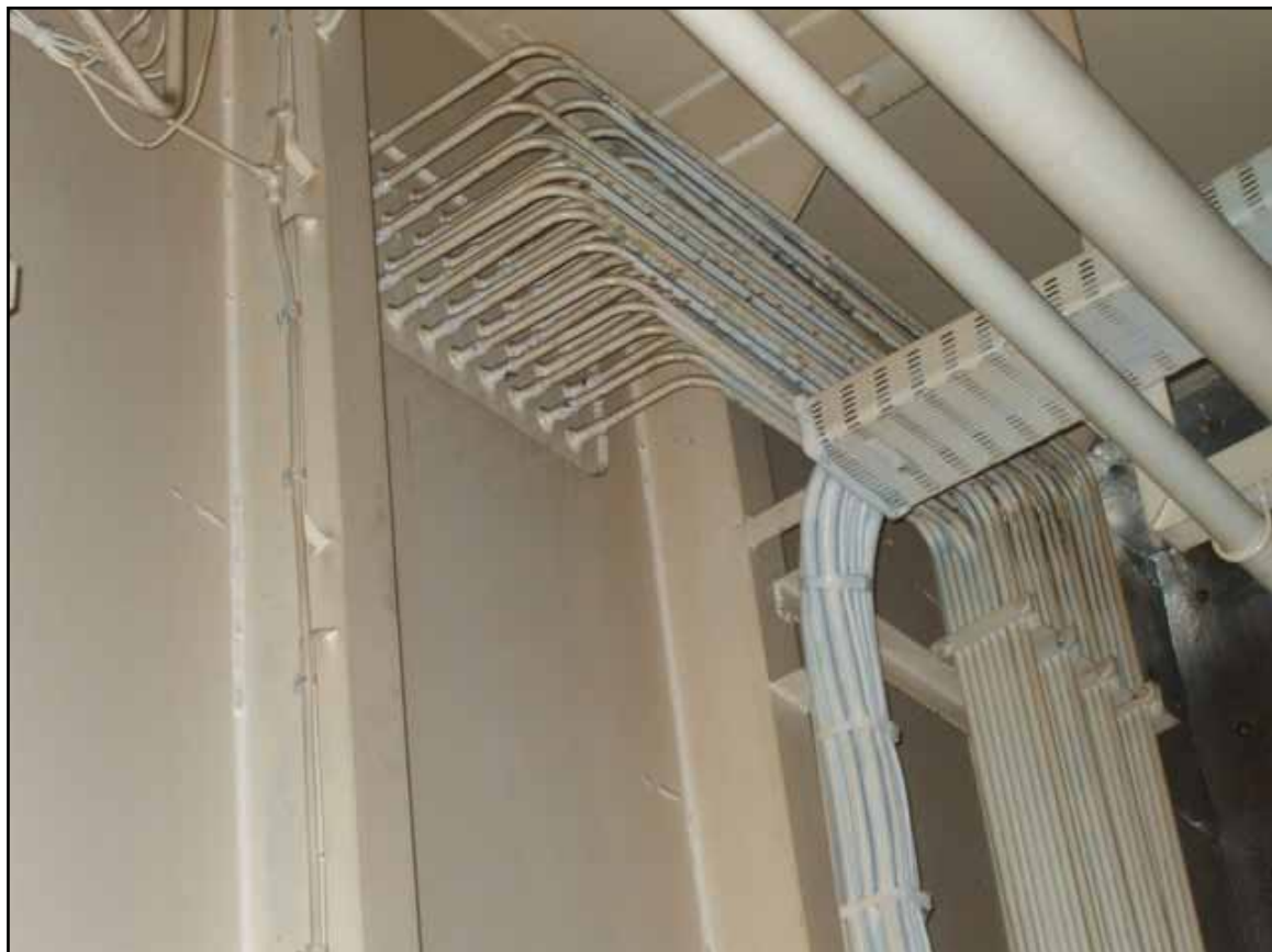
Water ballast tank valves - hydraulic distribution lines
