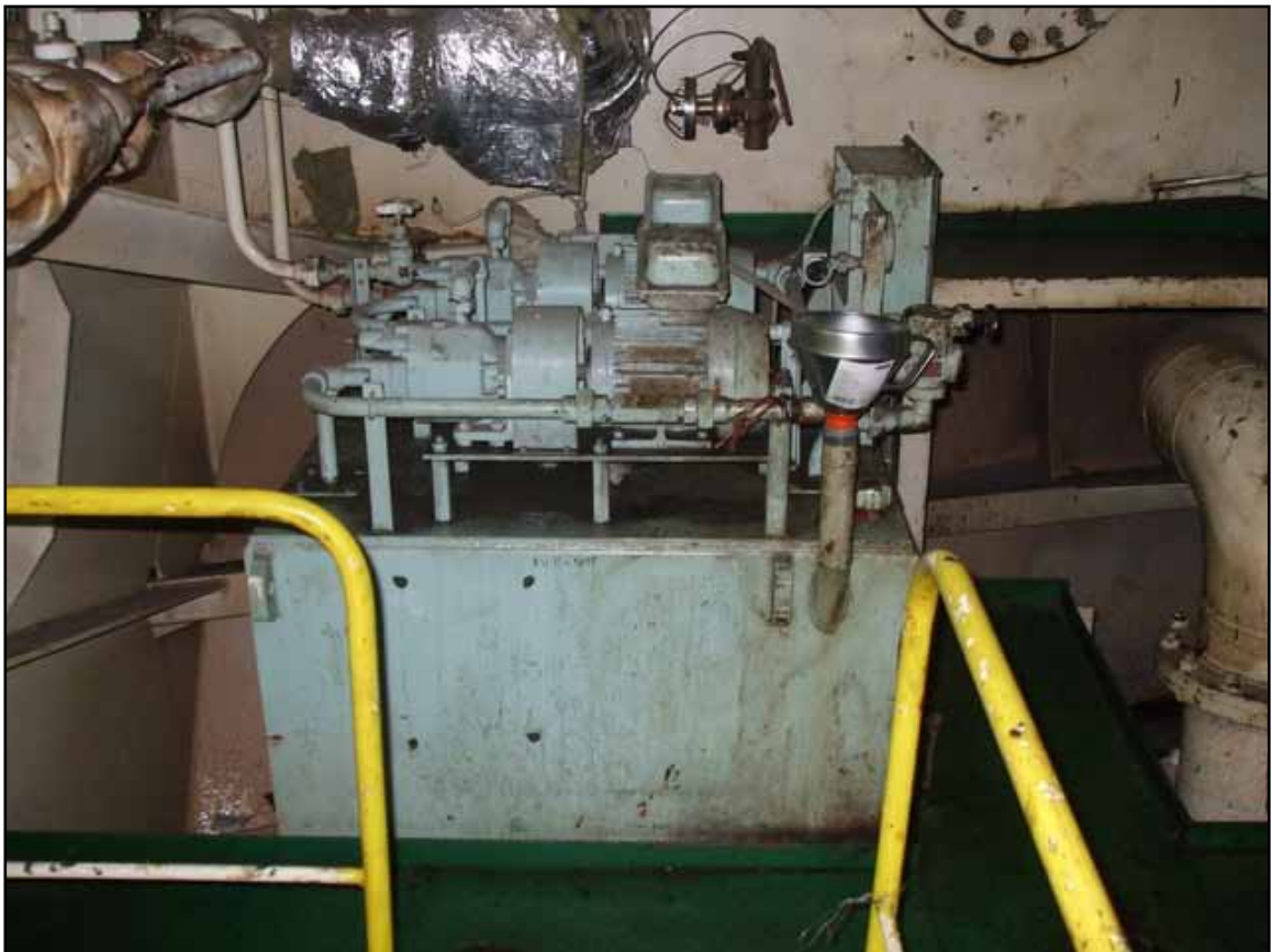
Water ballast tank valves - hydraulic power pack
