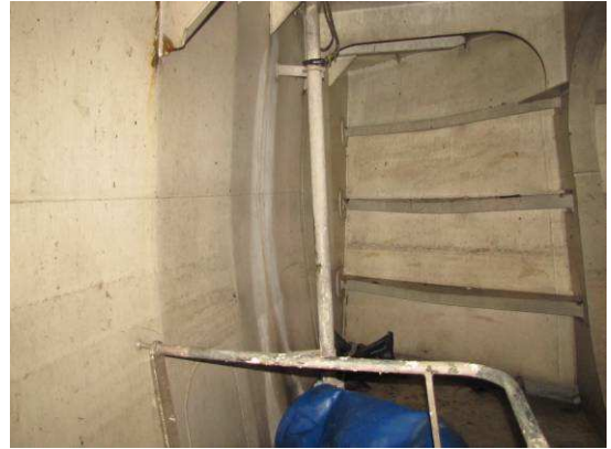
Aft bulkhead buckled towards the aft
