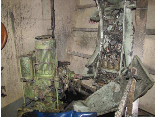
Emergency fire pump and electrical panel
