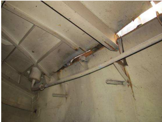
Top deck (Upper deck) inflated/broken
