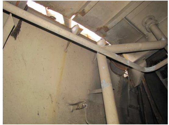
Top deck (Upper deck) inflated/broken
