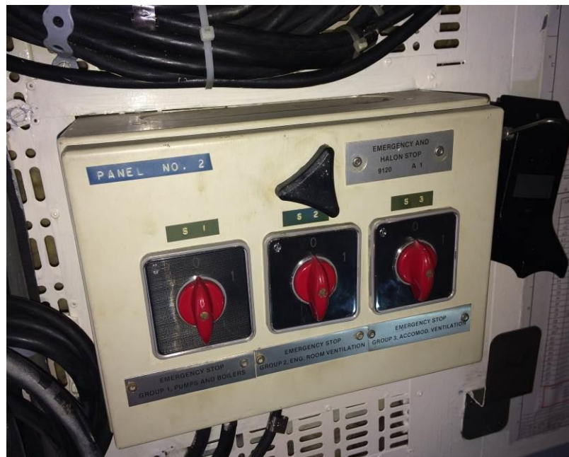
Figure 8: Emergency stops for pumps, boilers and ventilation
