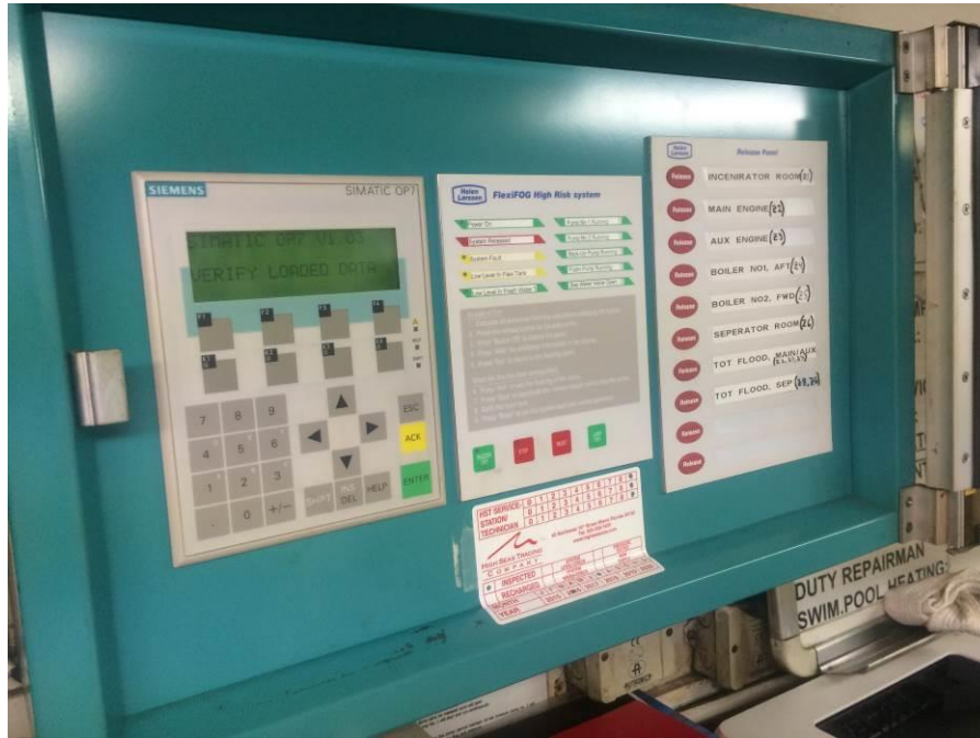
Figure 12: Flexifog system in ECR
