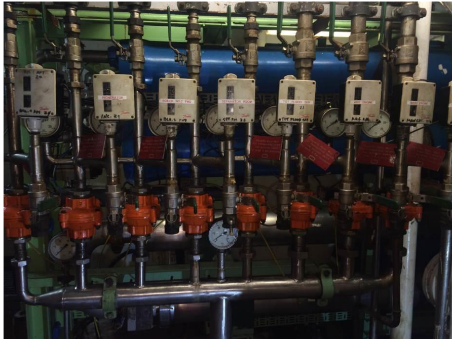
Figure 15: Water mist release solenoids in the pump room
