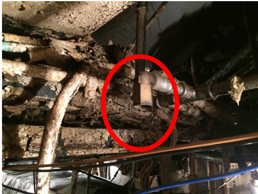
Figure 36: Showing missing nozzle in the high-risk zone.
