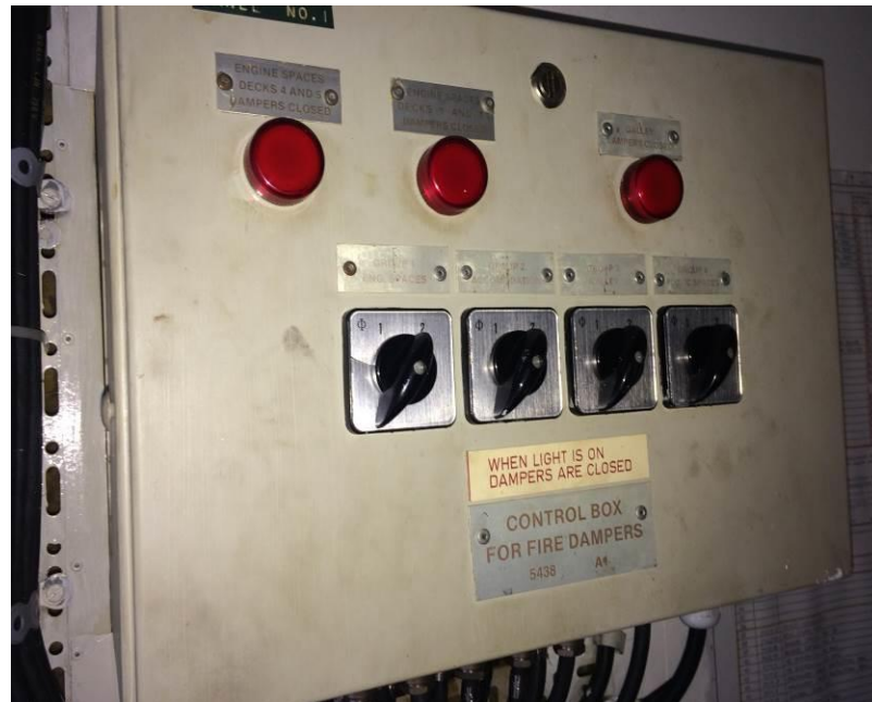
Figure 9: Control box for fire dampers
