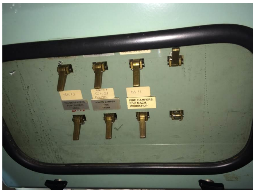
Figure 10: Damper controls
