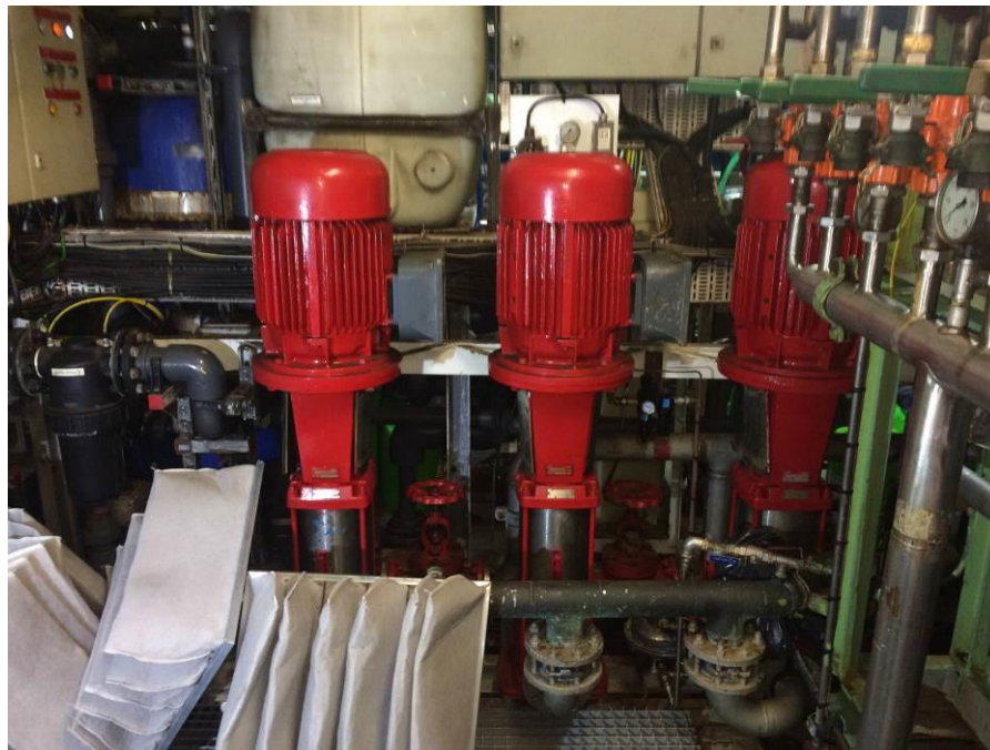
Figure 14: Water mist supply pumps in the pump room
