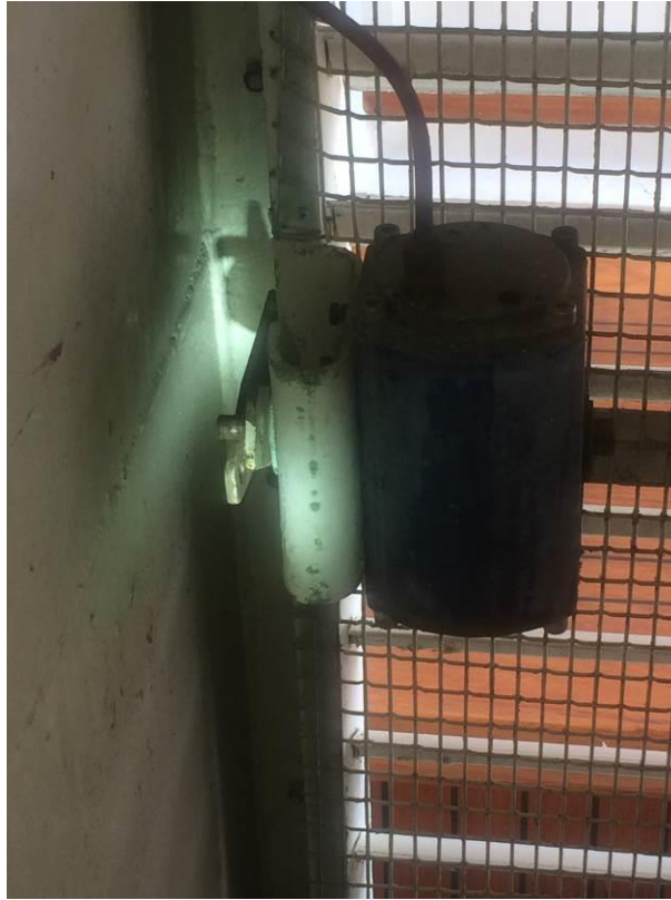
Figure 18: Air-actuated damper control for emergency generator
