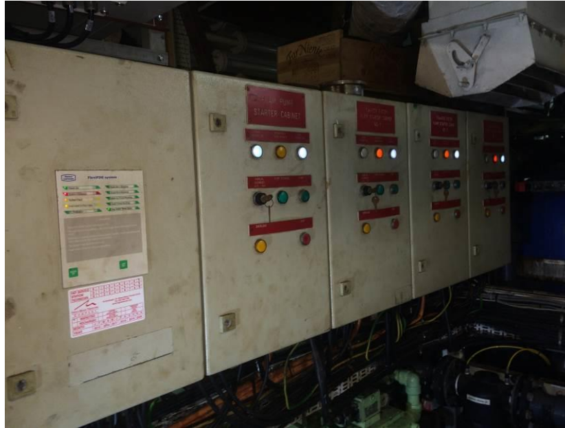
Figure 19: Sprinkler pump starters in the pump room
