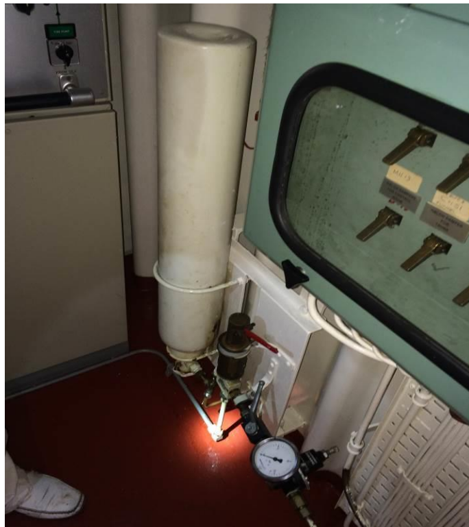
Figure 6: Emergency air reservoir and controls for Quick Closing Valves
