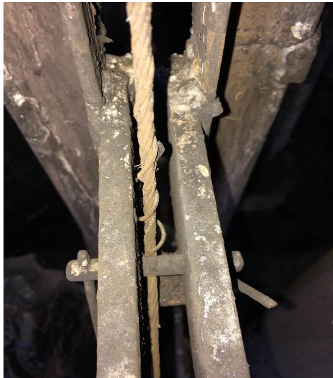
Figure 37: Frayed wire on hatch closing mechanism
