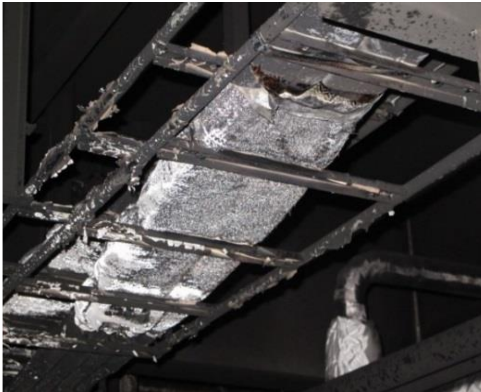
Figure 12: Damaged cables
