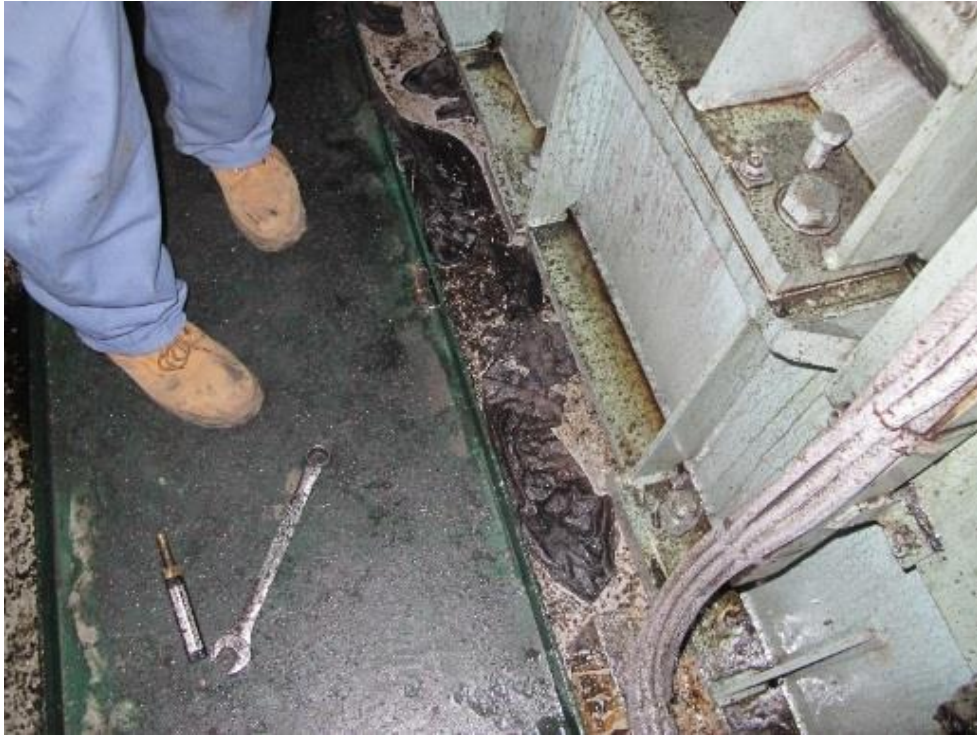
Figure 3: Replacement pocket, thermometer and spanner
