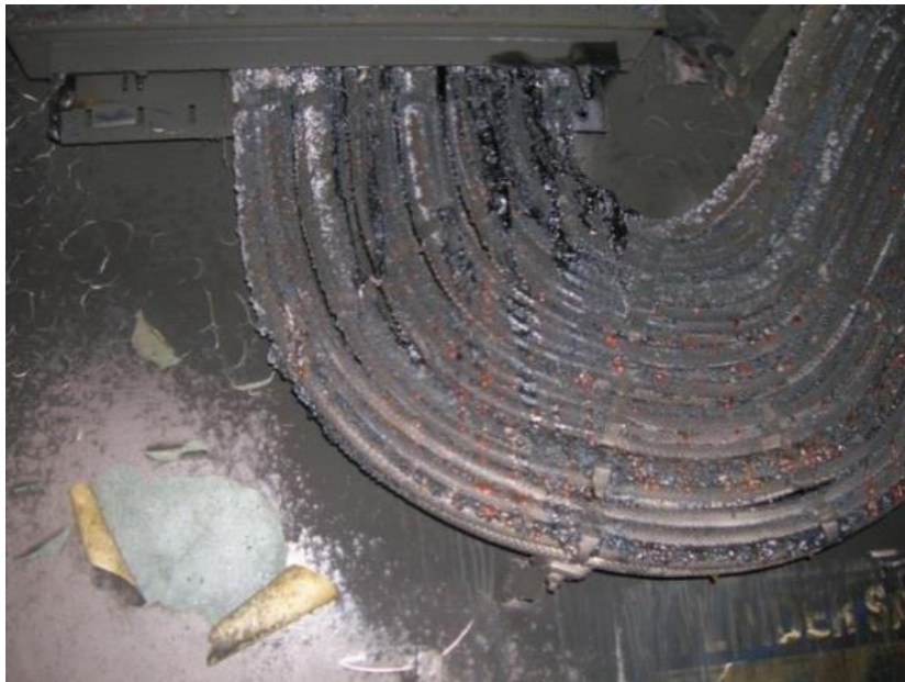
Figure 17: Damaged cables
