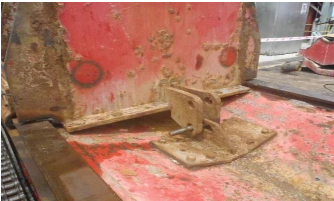
Figure 7: Riser support Fixed to Skate with a bolt (nut is not connected to the bolt)
