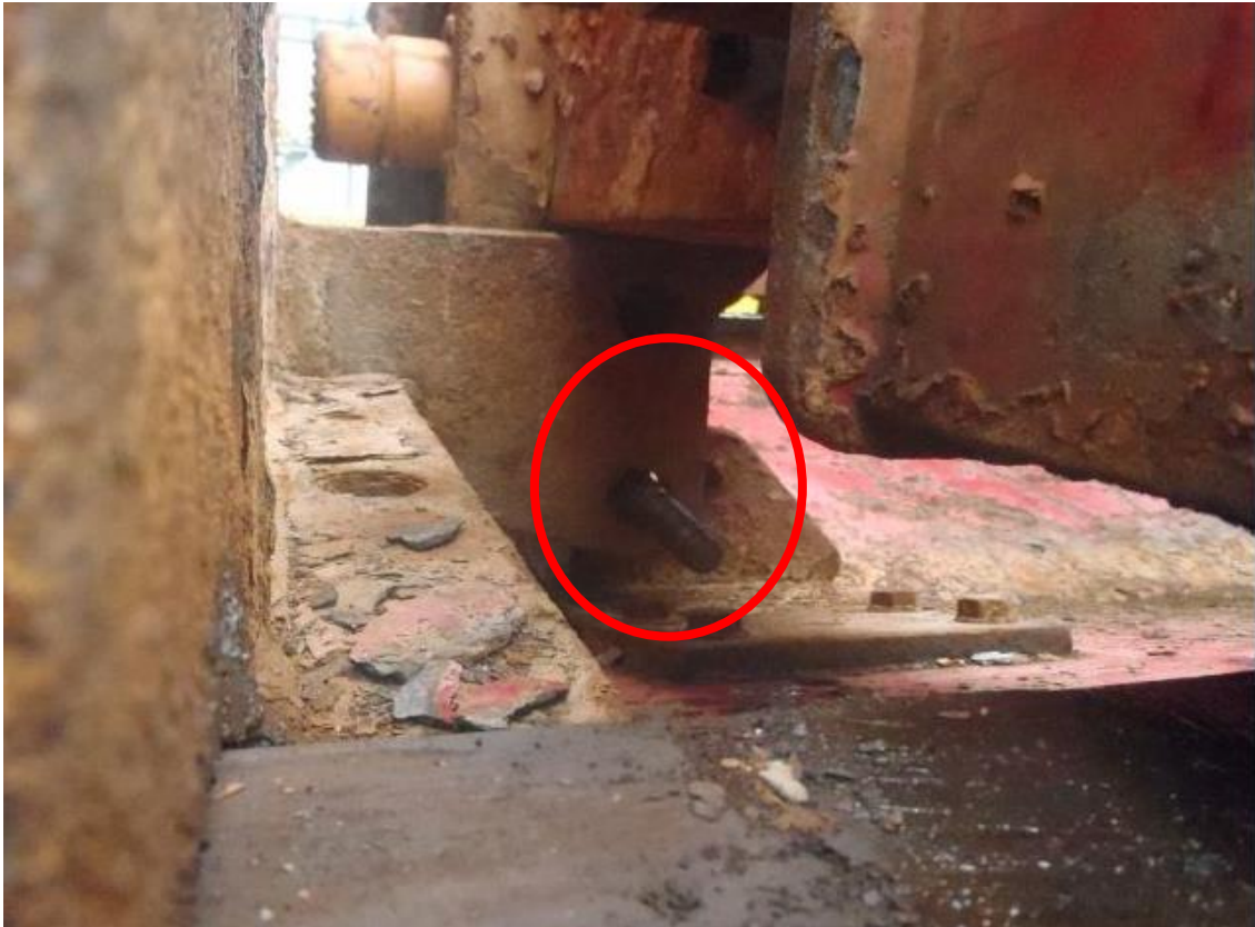
Figure 20: Riser support secured to the skate – bolt indicated without nut attached
