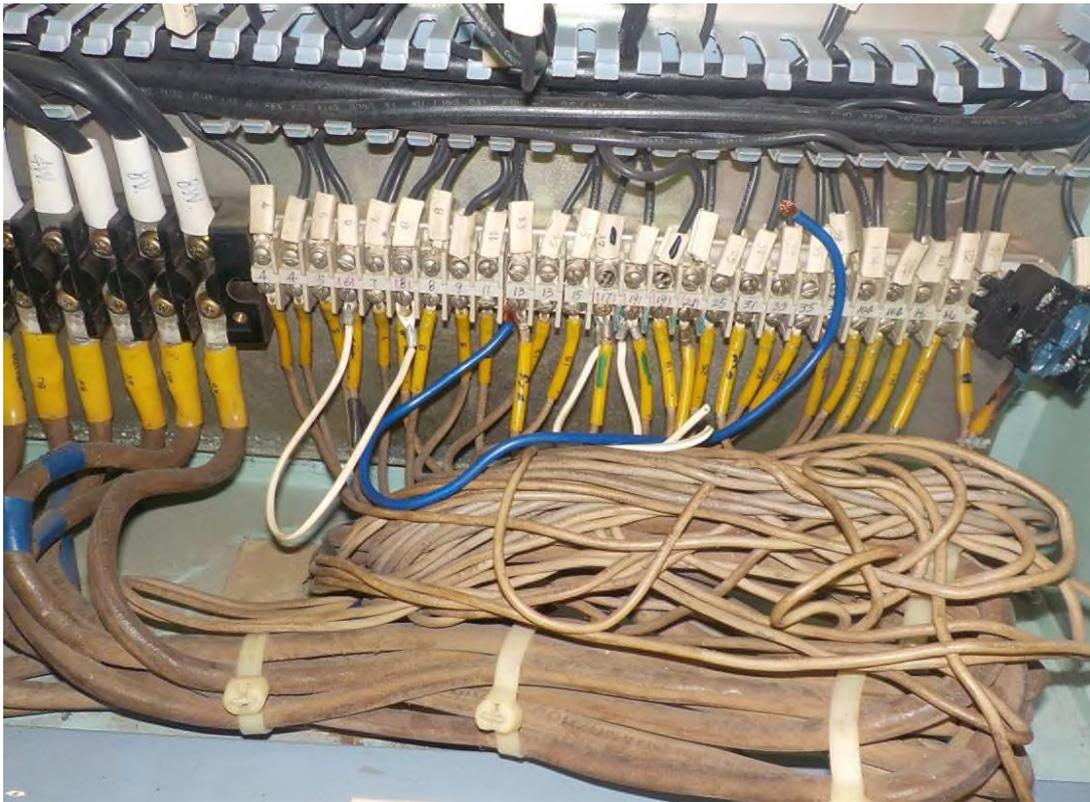
Figure 17: View of bypass connections within switchboard
