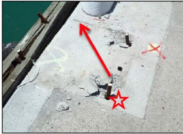
Figure 9 Bollard 26 after the failure, showing the direction of mooring lines to the ship
