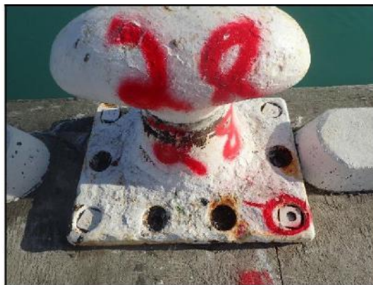
Figure 12 Underutilisation of the bollard securing arrangement
