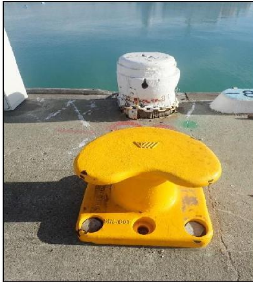
Figure 13 Newly installed steel bollard
