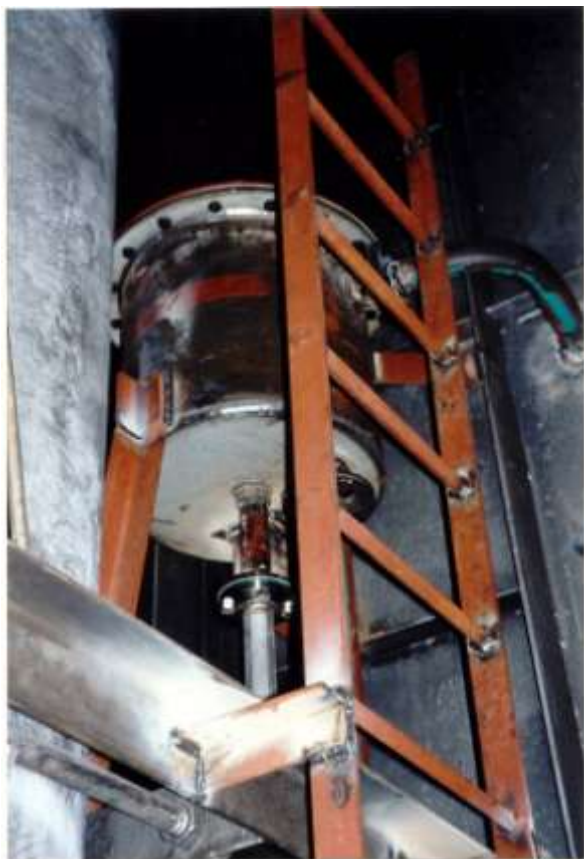
Photo. 3 New collection tank for deck hydraulic system reservoir tank vent pipe.
