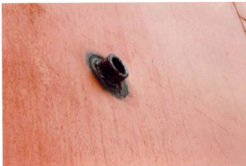
Photo.5 Deck hydraulic reservoir tank vent pipe collection tank vent through side of funnel.
